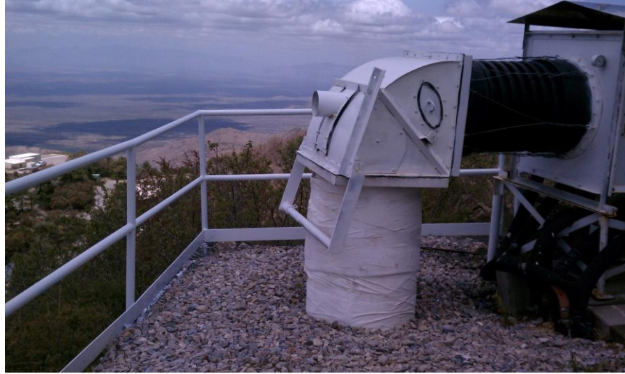
Figure 10. Guardrails installed around the shop heat exchanger.
