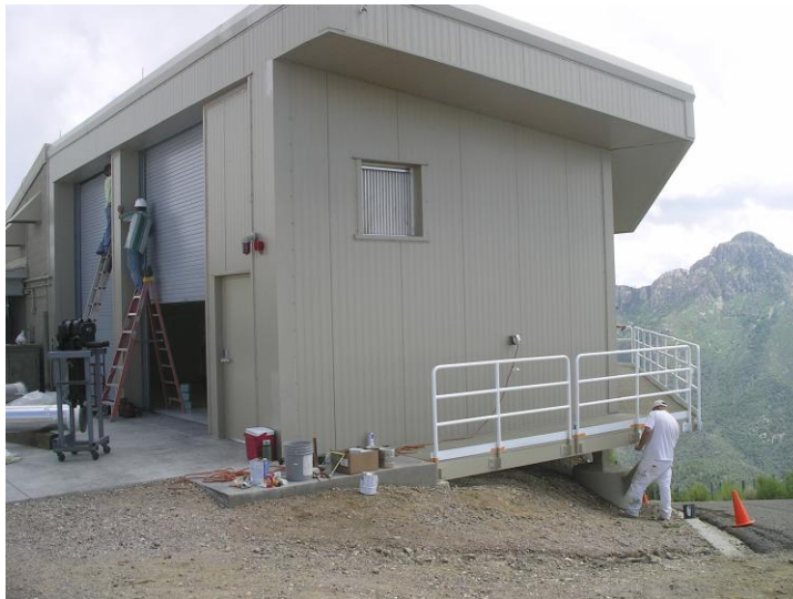
Final painting and door work on the Instrument Repair Facility.
