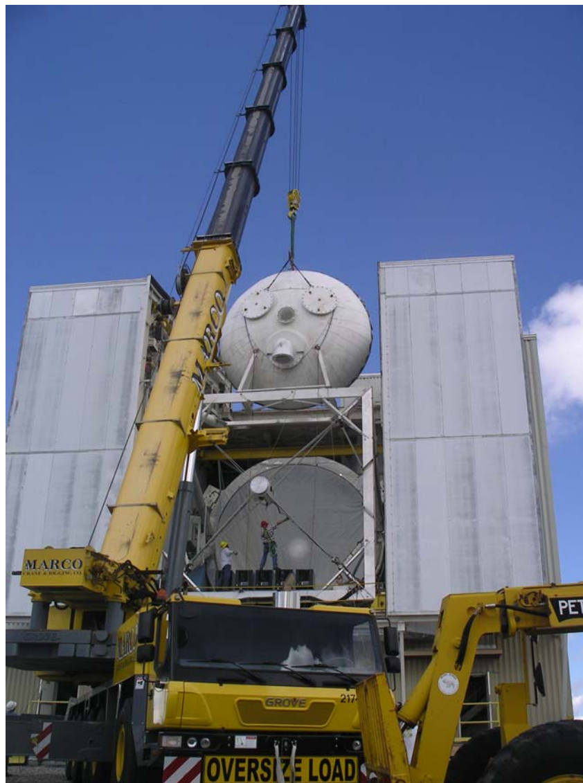
During summer shutdown: preparing to cover the MMT 6.5-m mirror with the vacuum bell jar prior to re-aluminizing the mirror.
