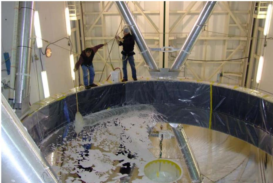
Figure 4: Brian Comisso and John Di Miceli complete wash of the mirror east side while the west (now clean) is being rinsed.
