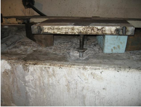
Old grout has been removed and the track reset.
