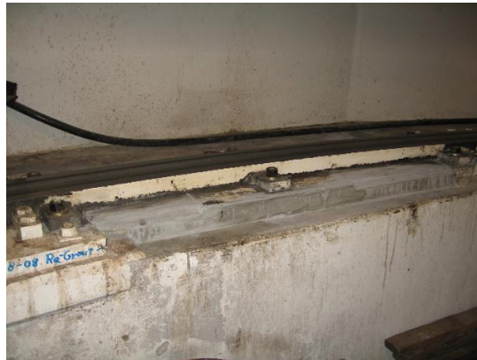
Grout is successfully placed; curing cycle is underway.
