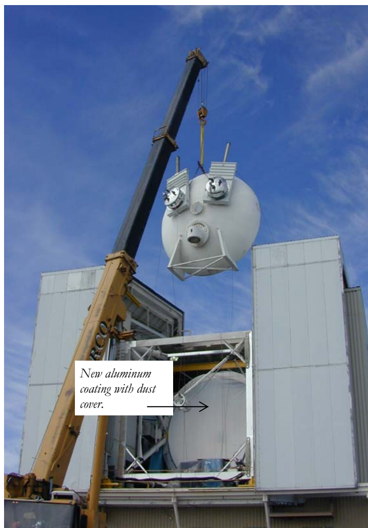
Removal of the vacuum head, with two cryogenic pumps and valves, following successful re-aluminizing of the MMTO 6.5-m primary mirror. Photo by Ken Van Horn (MMTO).
