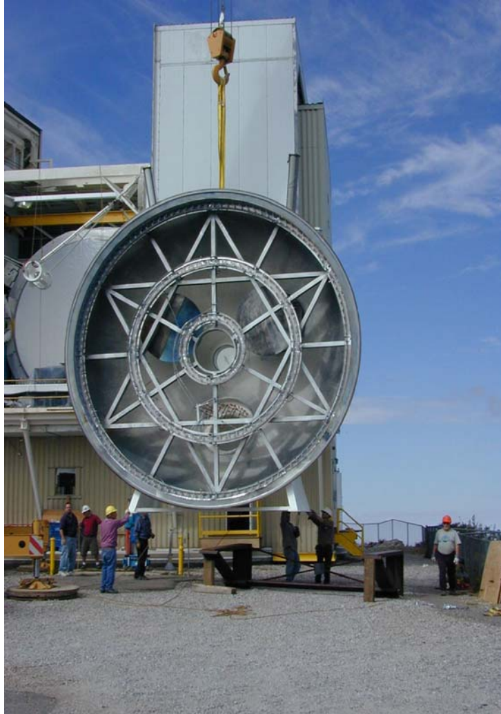
d) The vacuum head (belljar) is prepared for rotation to horizontal, and storage.
