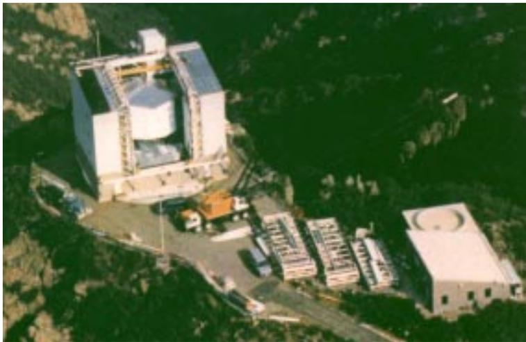
**FIGURE 6.** An aerial view of the MMT building modifications. The shutters are lying on the ground, and the slit is being enlarged. The telescope is cocooned with plastic tarp and a wooden top in order to protect it from the modifications and the monsoons. Also seen is the storage location for the primary mirror aluminizing chamber on the roof of the adjacent building. The modifications were completed in October 1995.
