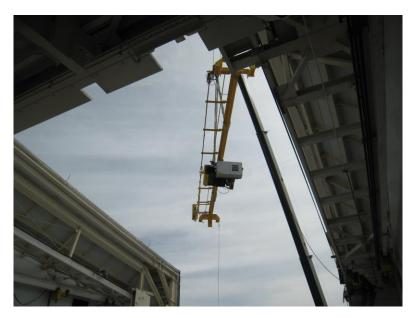
Moving the old 1978 bridge crane out of the chamber and the new 3-ton bridge crane into the chamber. For details, see page 18.
