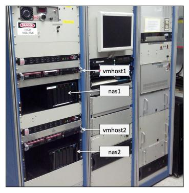
Figure 8. VM host computers and NAS devices in the "Server Room" (Room 3E) at the MMTO. The new hardware related to the "hacksaw" virtualization is labeled. Virtual host #1 ("vmhost1") and its associated network-attached storage device #1 ("nas1") are located above the similar vmhost2 and nas2. Power to vmhost1/nas1 is isolated from power to vmhost2/nas2 for additional safety and reliability. See text for more details.
